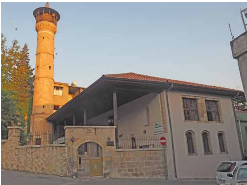
View 8.11 Hatuniye Mosque before the earthquake (2020)
