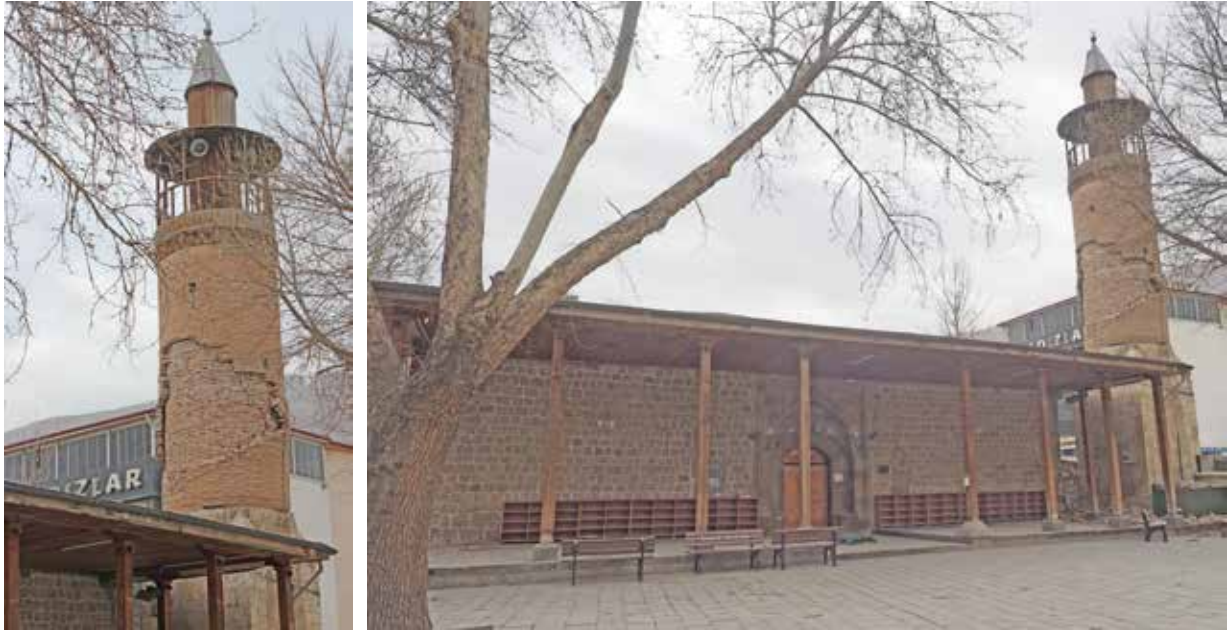
View 8.1 Elbistan Çarşı Atik (Alaüddeve) Mosque after the earthquake
