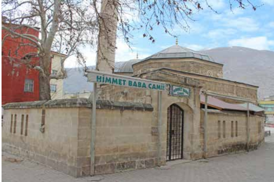
View 8.3 Elbistan Himmet Baba Mosque after the earthquake
