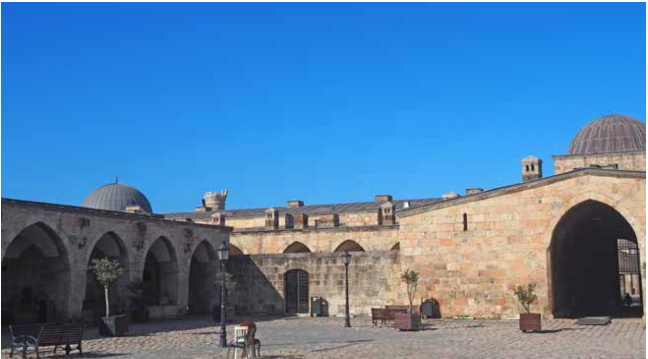
View 1.2 Payas Sokullu Mehmet Paşa Complex after the earthquake
