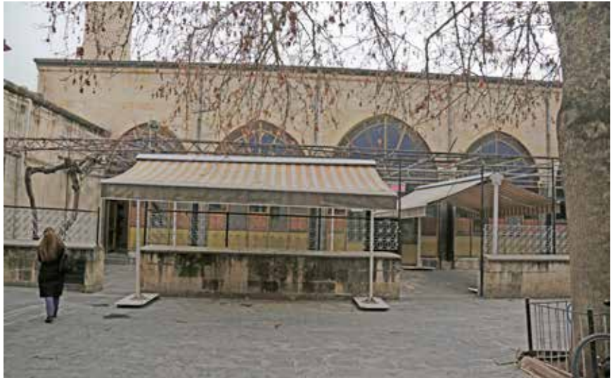
View 3.29 Hacı Veli Mosque after the earthquake
