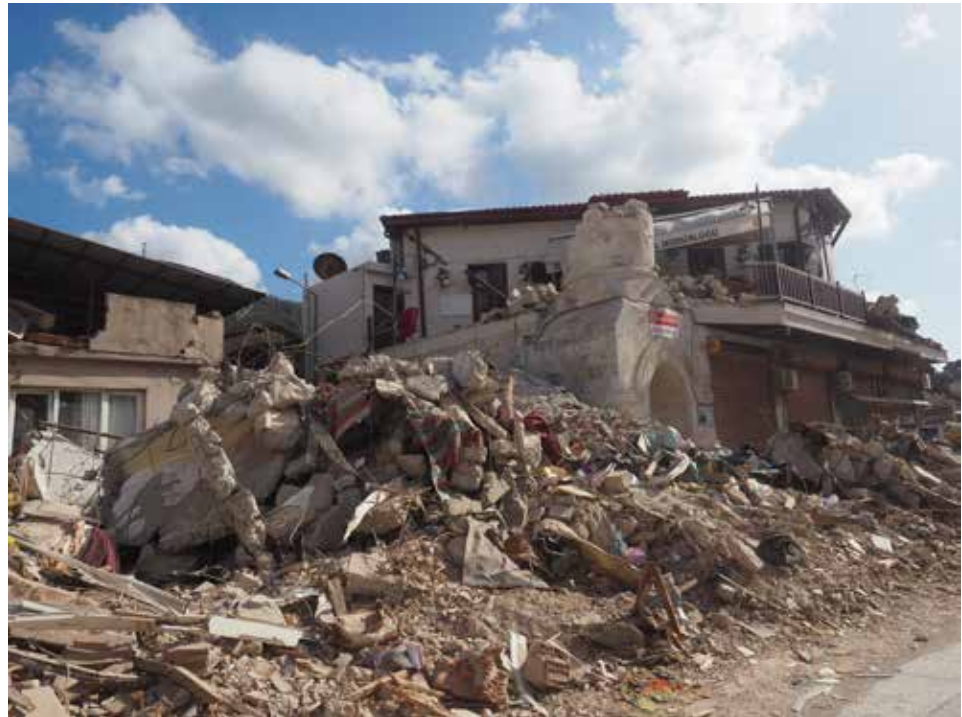
View 1.30 Şeyh Muhammed Mosque after the earthquake
