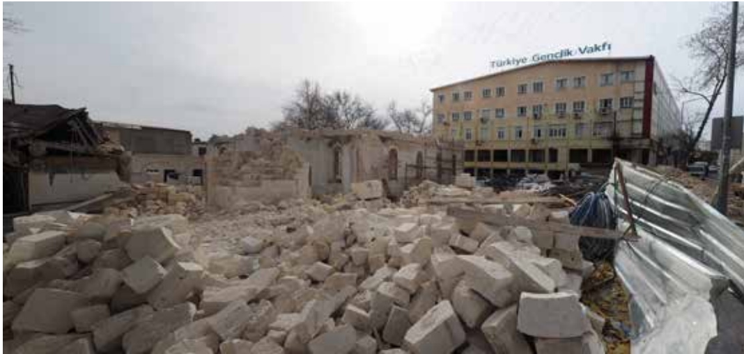
View 5.5 Çarşı Mosque after the earthquake
