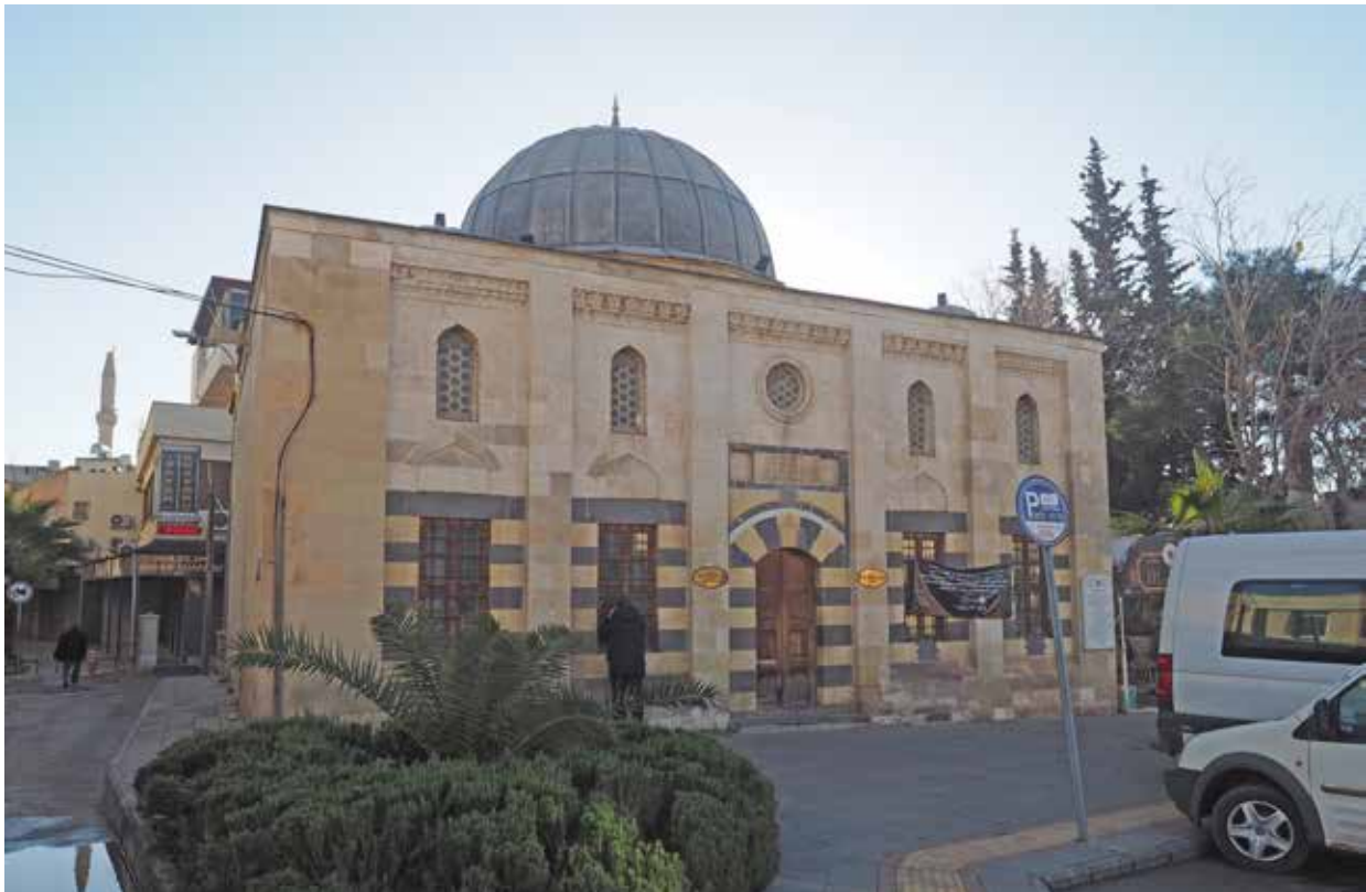
View 2.1 Mevlvihane Mosque after the earthquake
