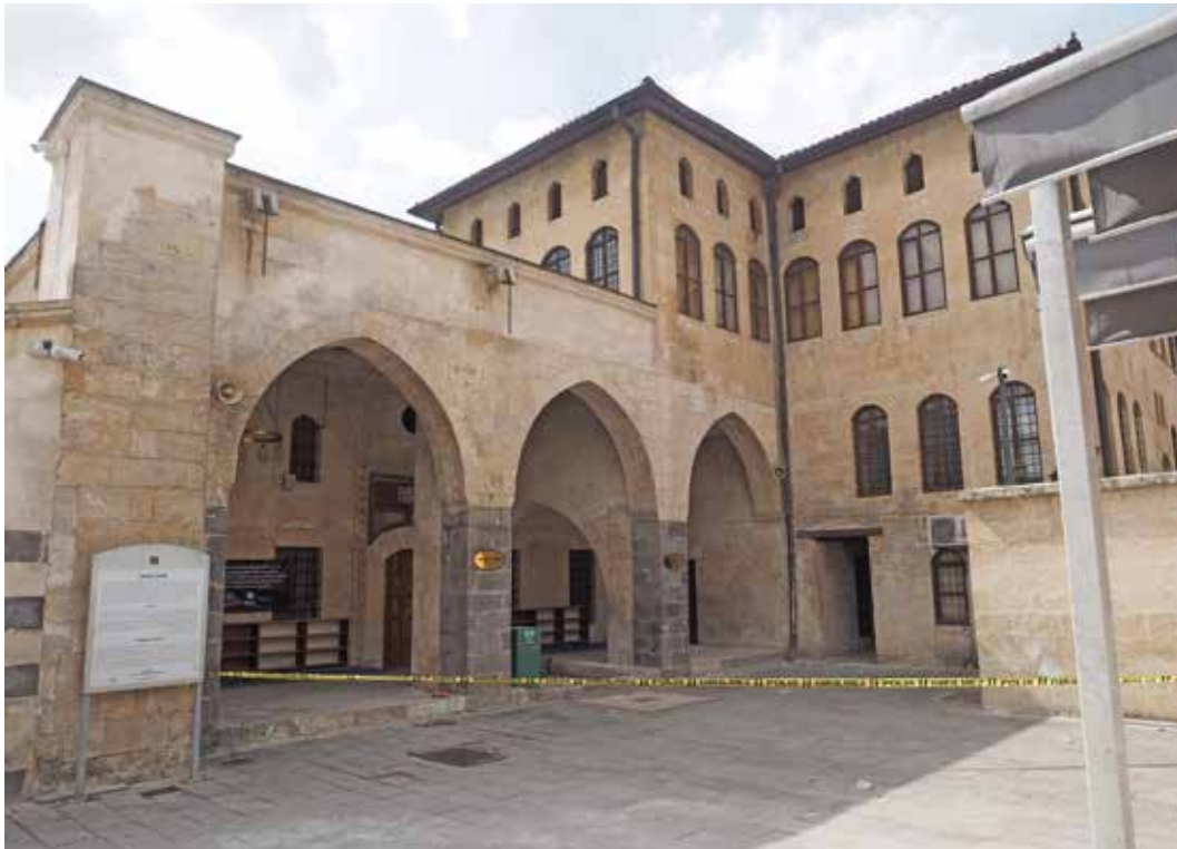
View 3.21 Tekke Mosque after the earthquake
