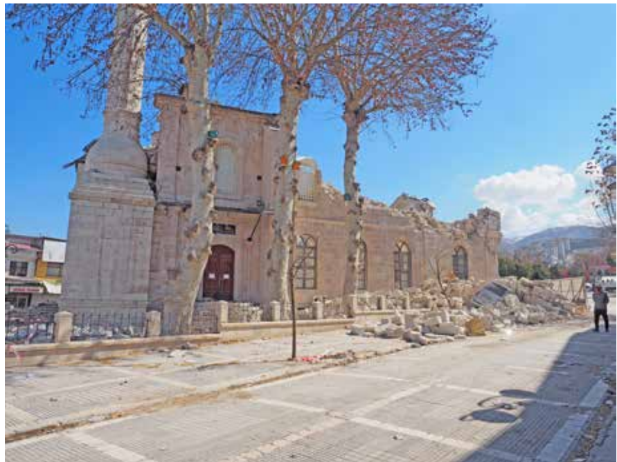
View 7.2 Yeni Mosque after the earthquake
