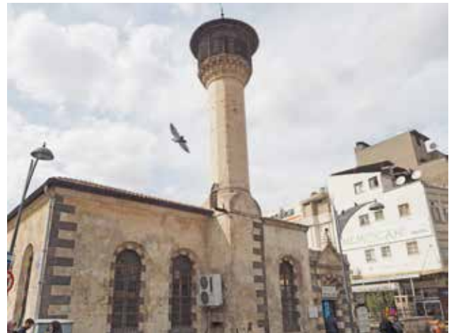
View 3.27 Hacı Veli Mosque after the earthquake
