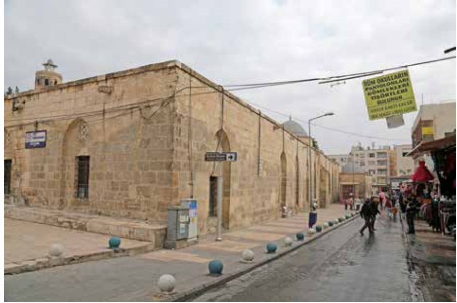
View 4.8 Ulu Mosque before the earthquake (2018)
