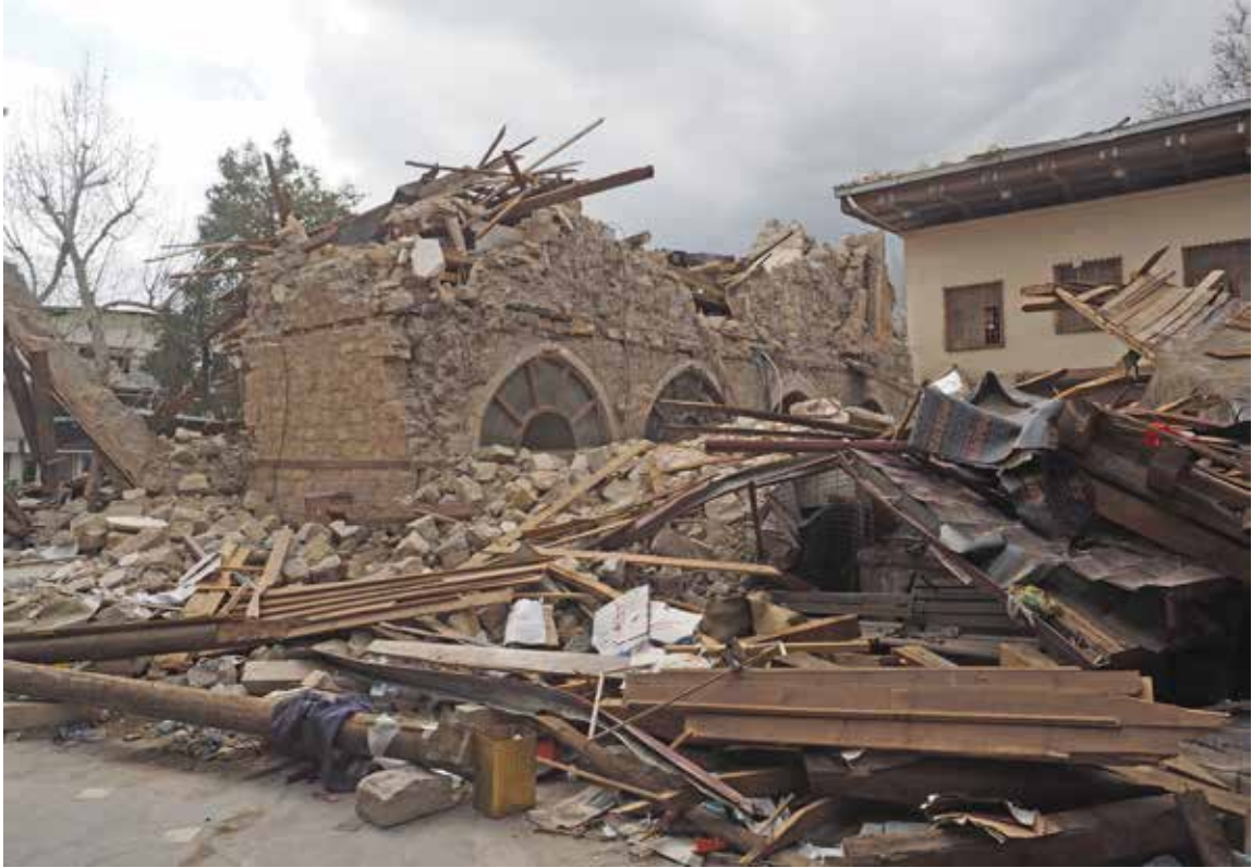
View 8.10 Saraçane Mosque after the earthquake
