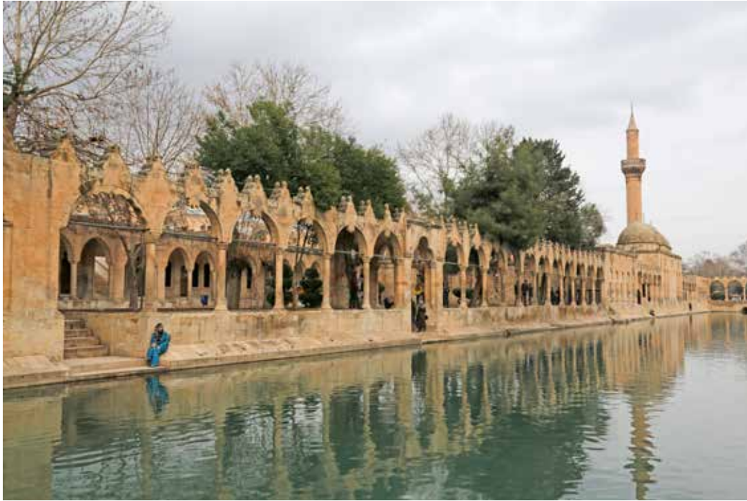
View 4.1 Rızvaniye Mosque before the earthquake (2018)
