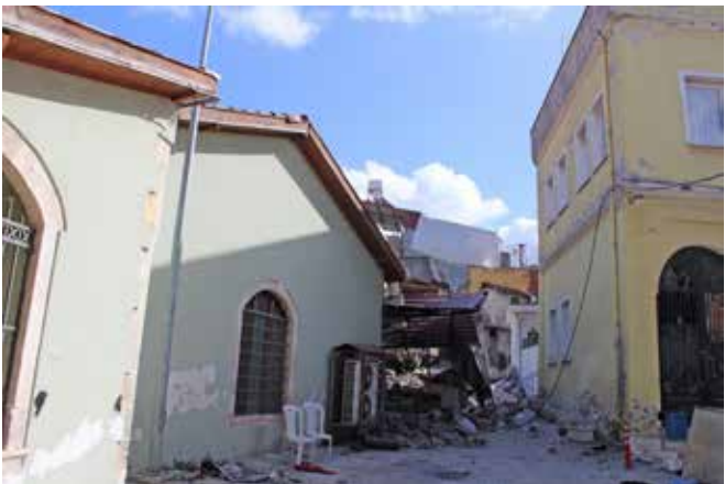
View 1.23 Ertuğrul Affan Mosque after the earthquake
