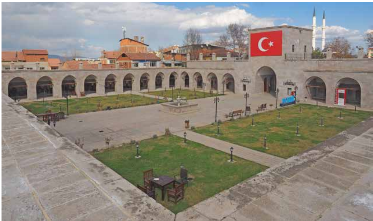
View 7.10 Silahtar Mustafa Paşa Caravanserai after the earthquake
