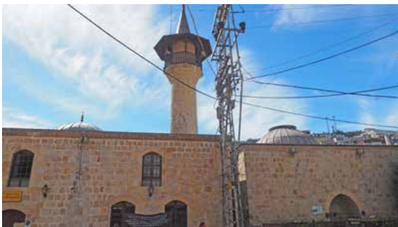
View 1.7 Belen Kanuni Sultan Süleyman Complex after the earthquake
