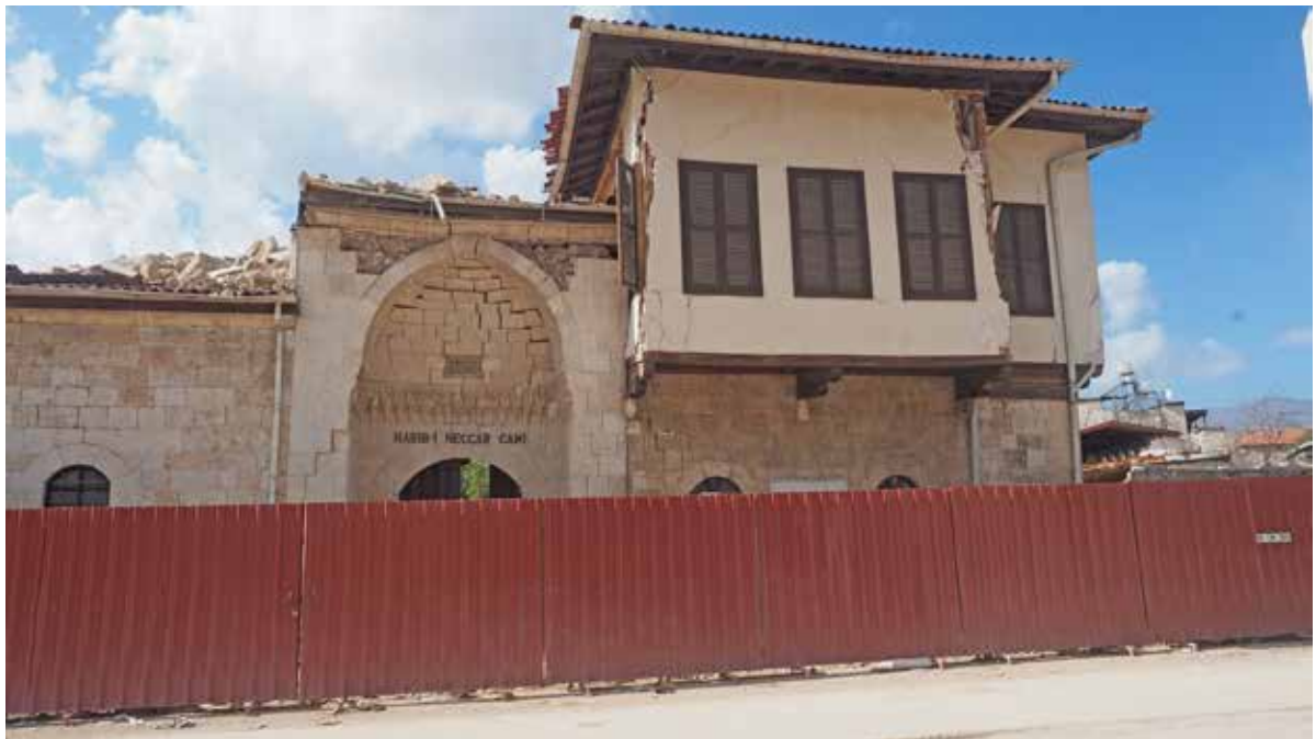
View 1.17 Habib-i Neccar Mosque after the earthquake
