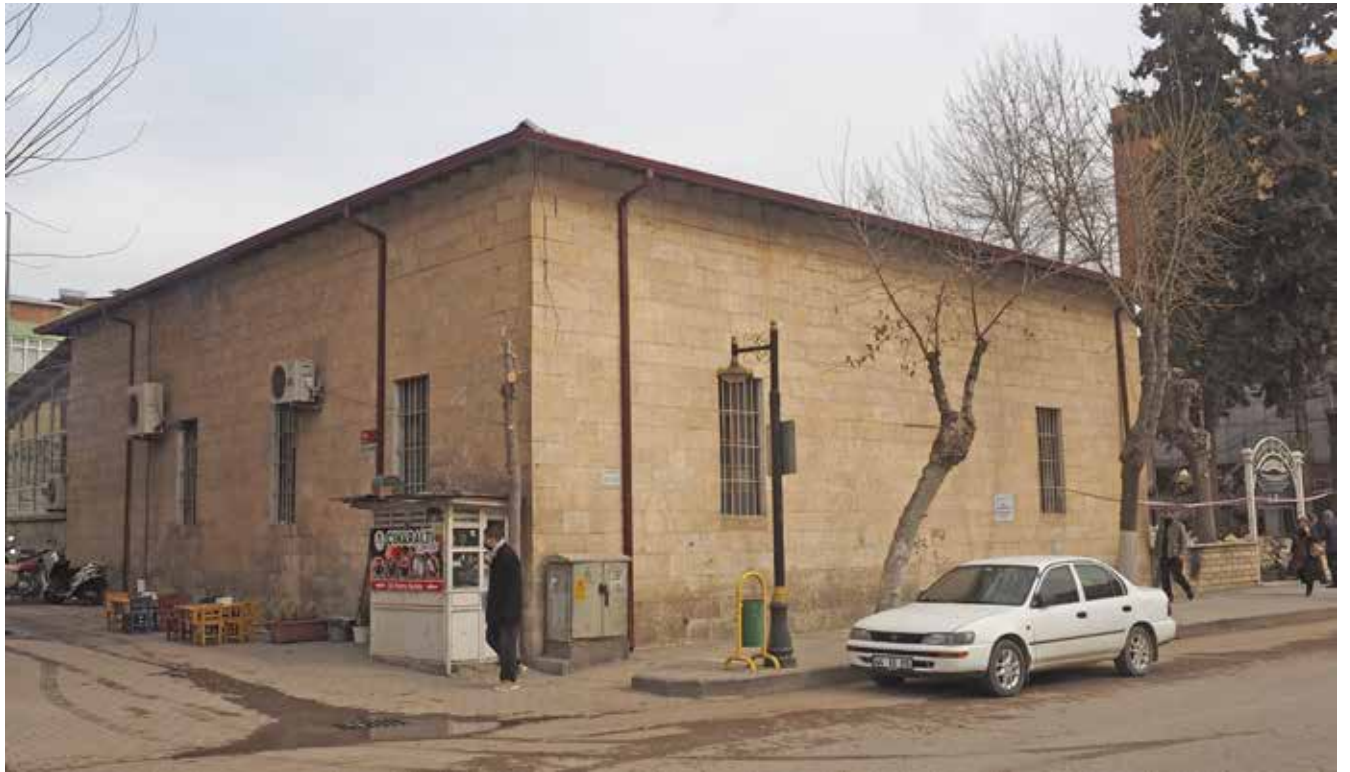
View 5.6 Eskişaray Mosque after the earthquake
