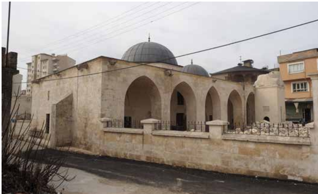
View 5.7 Musalla Mosque after the earthquake
