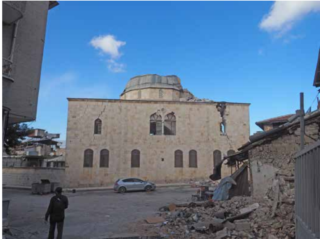
View 1.13 Şeyh Ali Mosque after the earthquake
