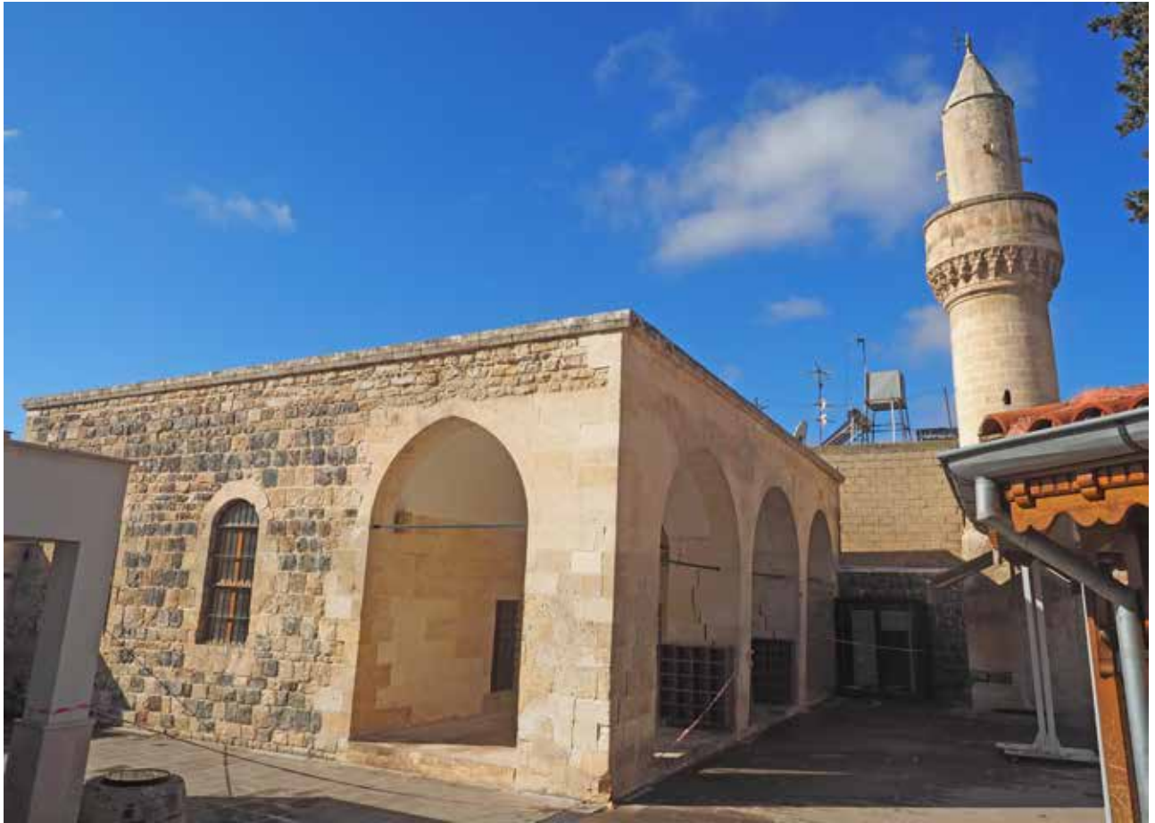
View 2.12 Pirlioğlu Mosque after the earthquake
