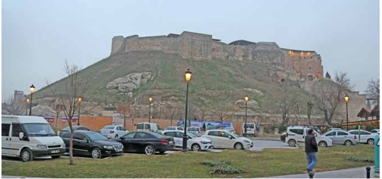
View 3.1 Gaziantep Citadel before the earthquake (2018)
