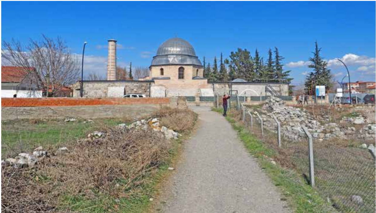
View 7.3 Battalgazi Ulu Mosque after the earthquake
