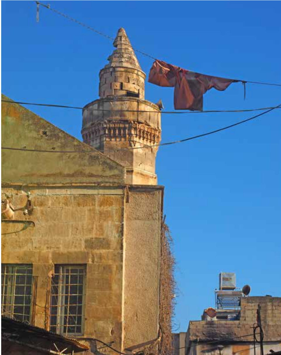
View 2.2 Şihlar Mosque after the earthquake
