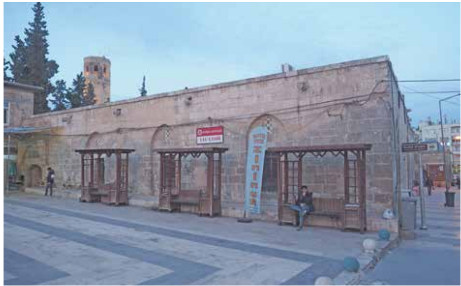
View 4.9 Ulu Mosque after the earthquake
