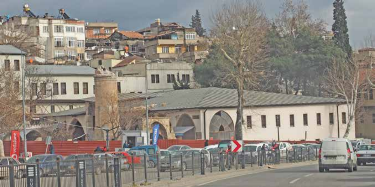
View 8.9 Kahramanmaraş Ulu Mosque after the earthquake
