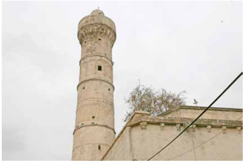
View 4.6 Dabakhane Mosque before the earthquake (2018)
