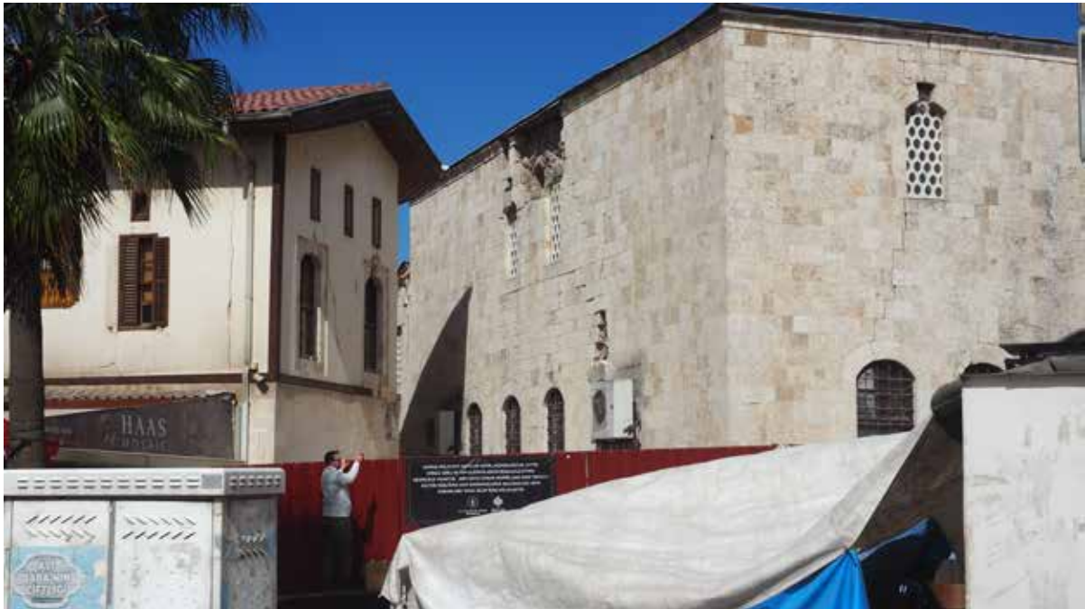
View 1.18 Habib-i Neccar Mosque after the earthquake
