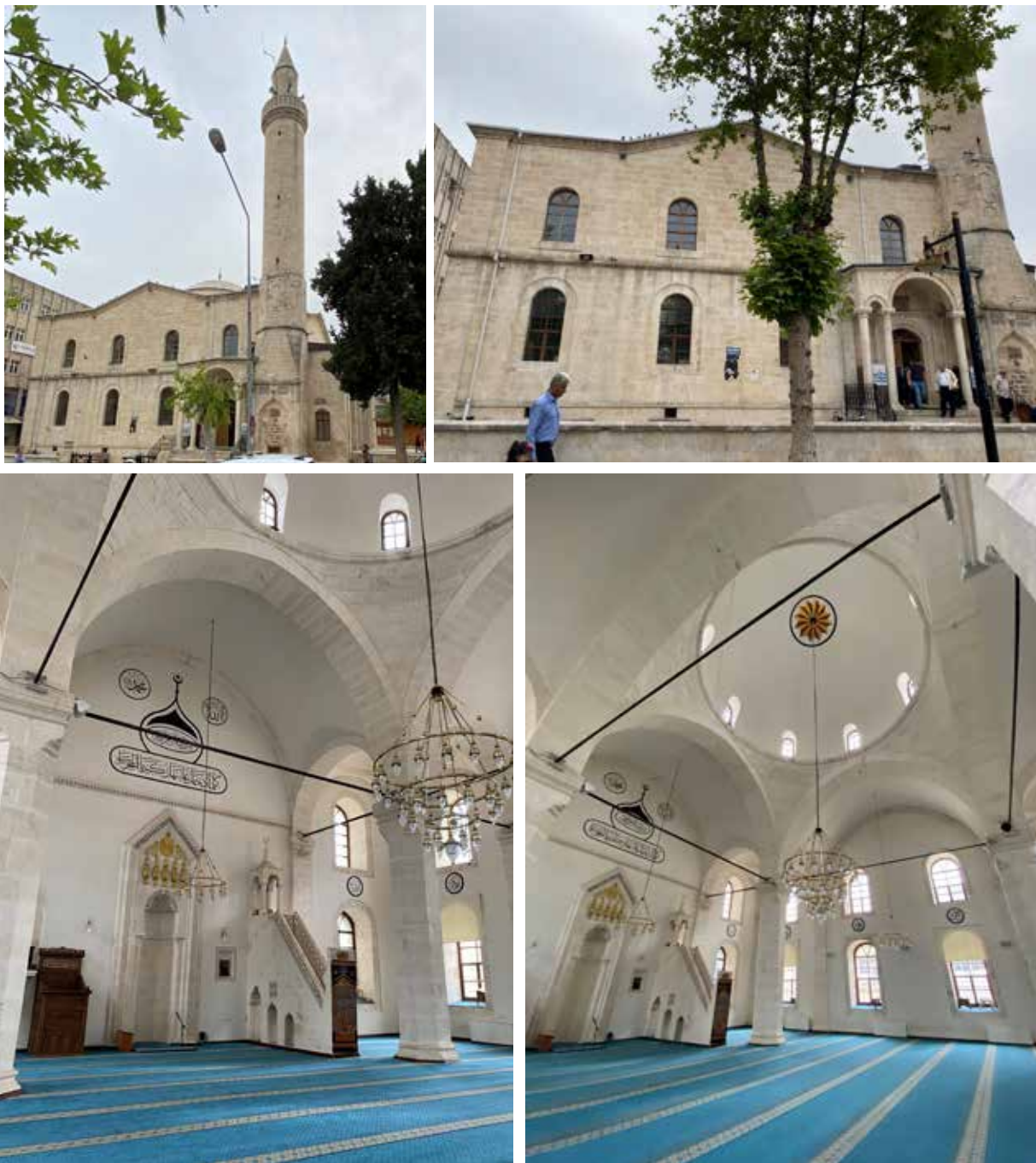
View 5.1 Adıyaman Ulu Mosque before the earthquake (2022)
