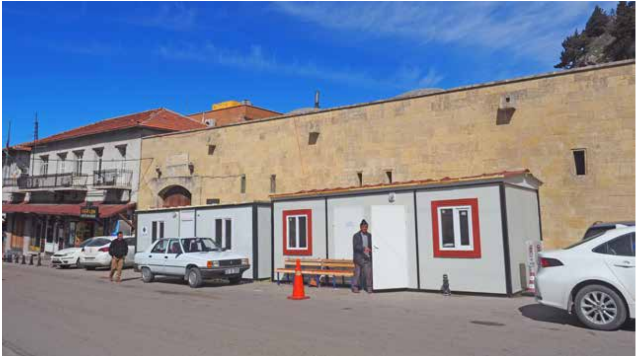
View 1.8 Belen Kanuni Sultan Süleyman Complex after the earthquake
