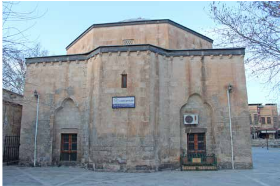
View 4.4 Mevlvihane Mosque after the earthquake
