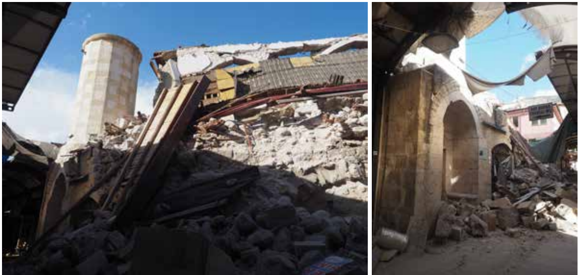
View 1.28 Mahremiye Mosque after the earthquake
