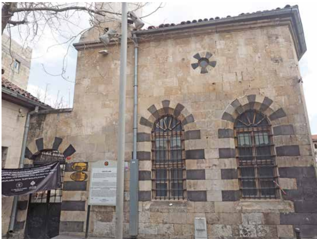
View 3.22 Kozluca Mosque after the earthquake
